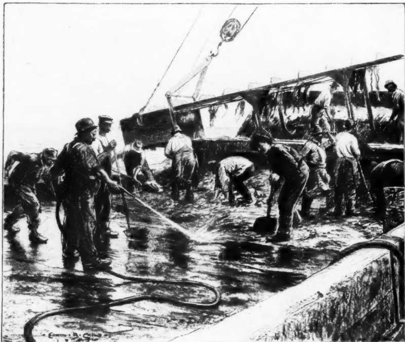
Unloading garbage with metal belt conveyor from scows at Barren Island. Cleaning the deck of a scow after unloading.
